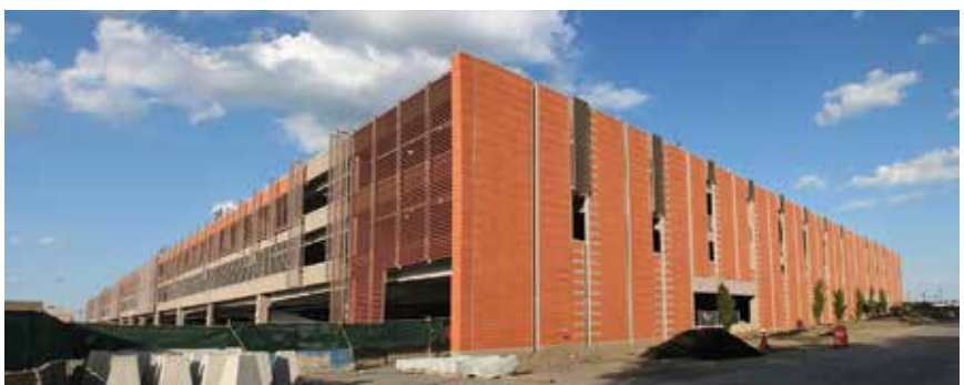
The Consolidated Rental Car Facility (CONRAC) at Logan International Airport in Boston, Mass., features the first use of terra-cotta embedded into structural precast concrete panels. Photos: Fennick McCredie Architecture.
