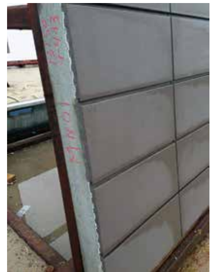
Terra-cotta was embedded into the precast concrete architectural walls used to clad the Hyatt Regency expansion at Tysons Corner in McClean, Va. A custom frame was designed to cover the edges of panels at window openings to avoid the necessity of returns on panels. Photos: RTKL Associates.
