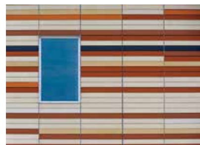
Terra-cotta was embedded into insulated precast concrete panels at the University of Missouri's Henry W. Bloch Executive Hall for Entrepreneurship and Innovation in Kansas City, Mo., when designers found it was more economical than cladding a rainscreen. Photos: Jacia Phillips Photography.
